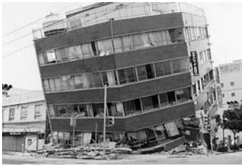
Photo.14. 阪神大震災で倒壊したビル。A building which was crushed by Great Hanshin-Awaji Earthquake.
